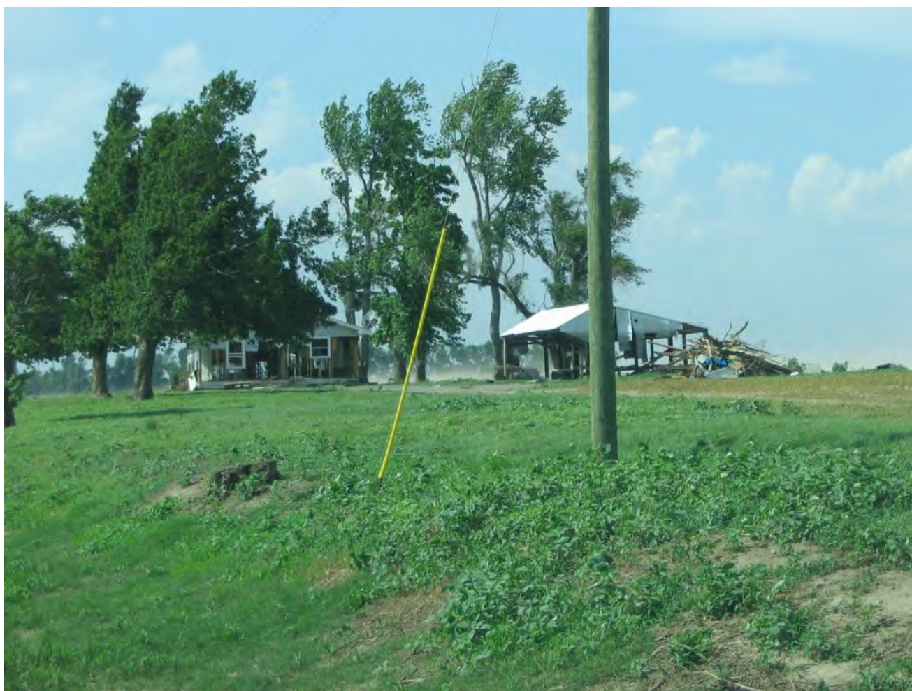
Figure 2. Flood damage buildings. A house and shed located in New Madrid floodway that was damaged by 3 to 5 ft. of rapidly flowing floodwater from the Birds Point levee breach
