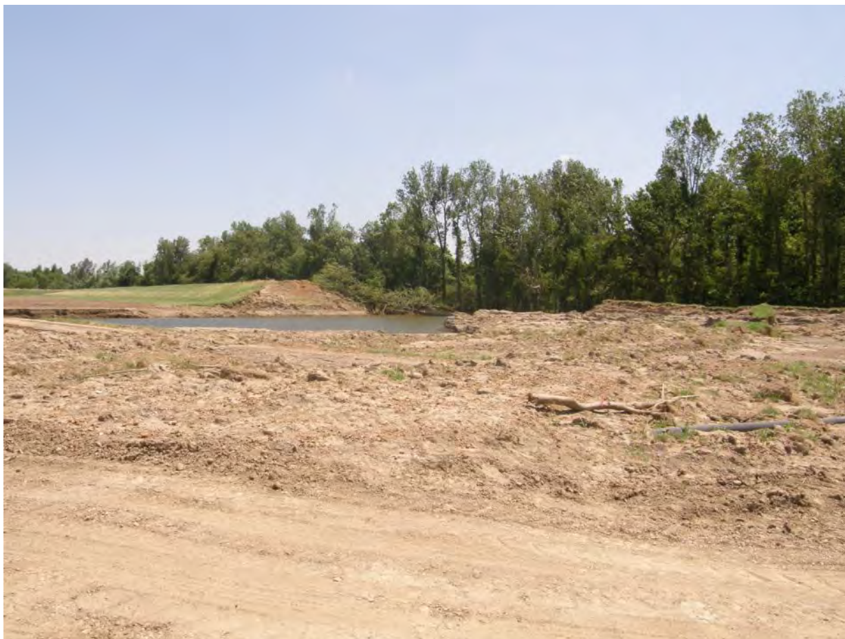
Figure 1. Birds Point levee breach. The Birds Point levee is showing the site of the first explosion is visible with remnants of the fuse plug levee and the crater lake extending into the adjacent agricultural lands that are still under floodwaters.
