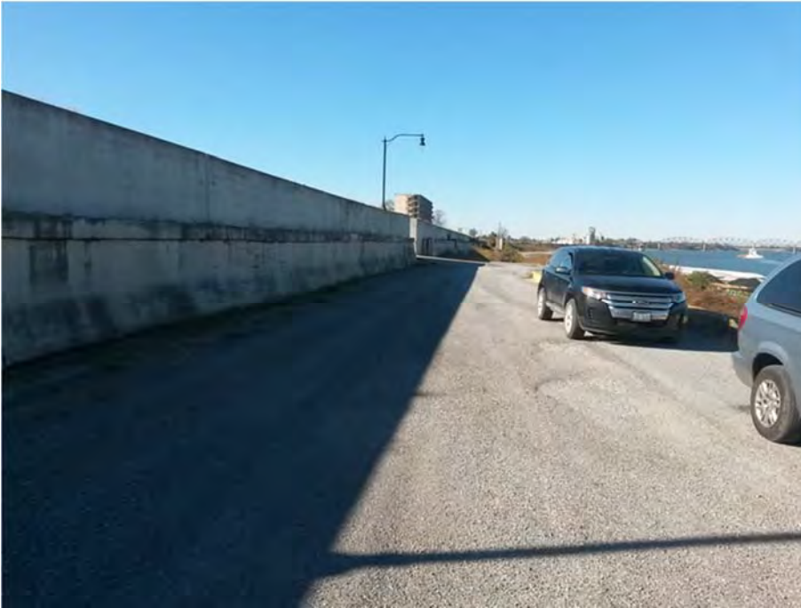
Figure 6. The Cairo, Illinois floodwall, built after the Great Flood of 1927, protects this city along its east side from the Ohio River.
