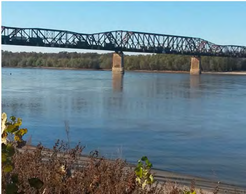
Figure 1. Railroad bridge over the Mississippi River at Thebes, Illinois. The bridge was built in 1905. The river valley is narrow (about 2000 feet wide) and the channel is lined with bedrock at this location: an excellent spot for a bridge.
