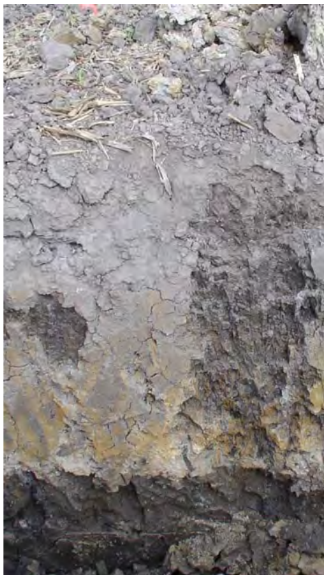
Practice Pit - 40 to 60 inches of Peoria and Roxana/lacustrine silts over Sangamon paleosol.
