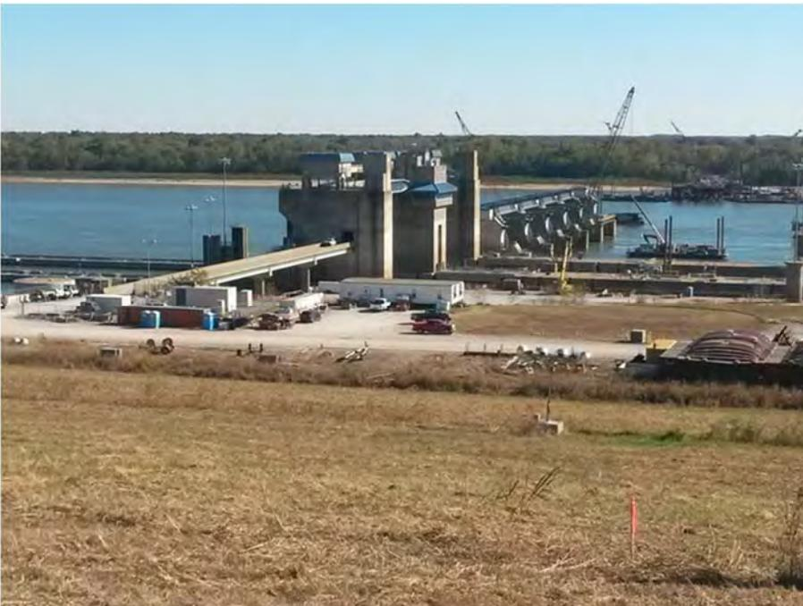
Figure 5. The Olmstead Lock and Dam on the Ohio River. This \$2.9 billion project was started in 1995 and is scheduled for a 2020 opening. Completion of this structure along with the removal of two sets of locks and dams upstream will reduce navigation time on the lower Ohio River by 3 hours.
