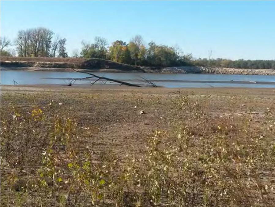
Figure 4. Breached levee. This breach occurred in January 2016 and is about one mile in length. Rip rap to the right of the levee breach was subsequently placed as a “repair”, but only covers a portion of the breach.
